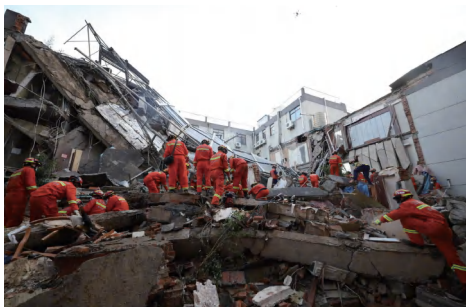
The site of the collapse
